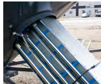
Slide Retro Rocket through manhole
