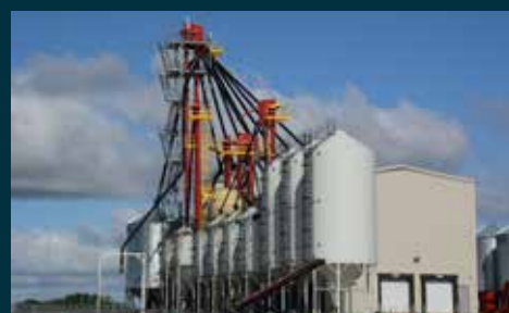
CLEANING & PROCESSING PLANTS
